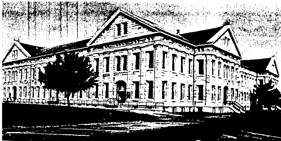
Figure 5. Original Stone Shop D (now Building 62), circa 1875. (RIA National Register of Historic Places Nomination Form, June 1987).
