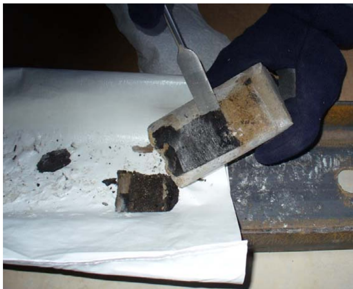
Figure 2-14 Removal of Expansion Joint Material (EJM)
