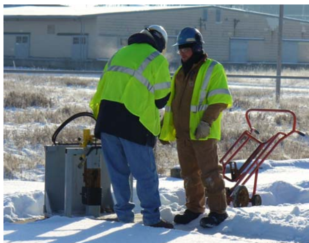
Figure 2-7 Concrete Core Sampling Team
