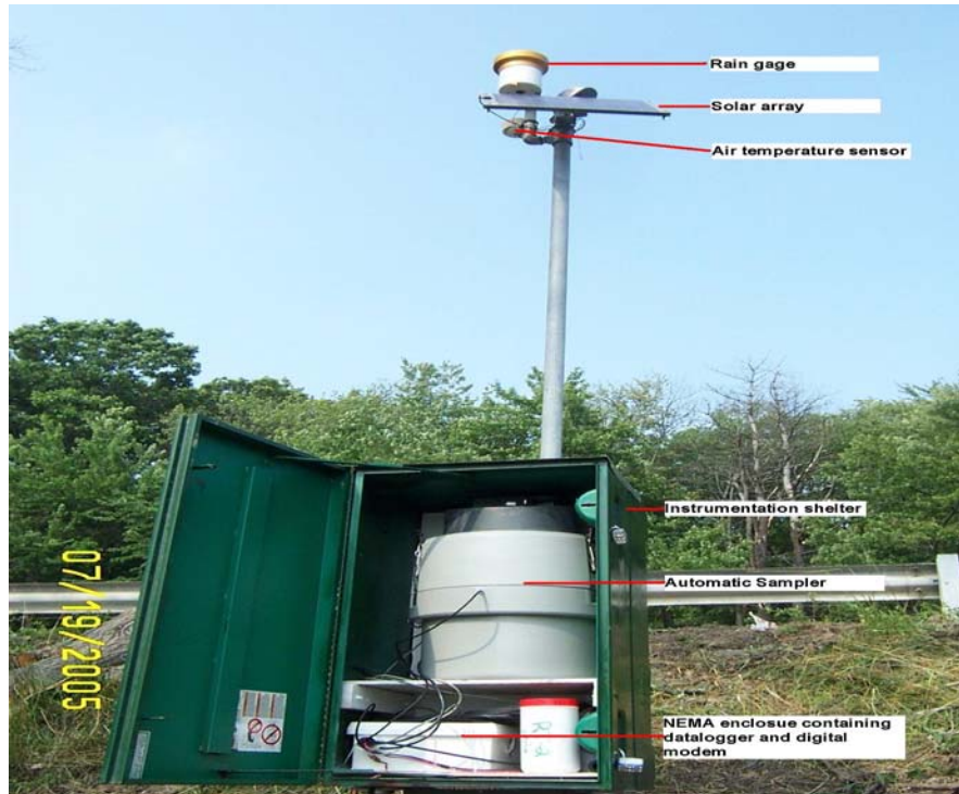
A. Anatomy of a Typical Highway Monitoring Station
