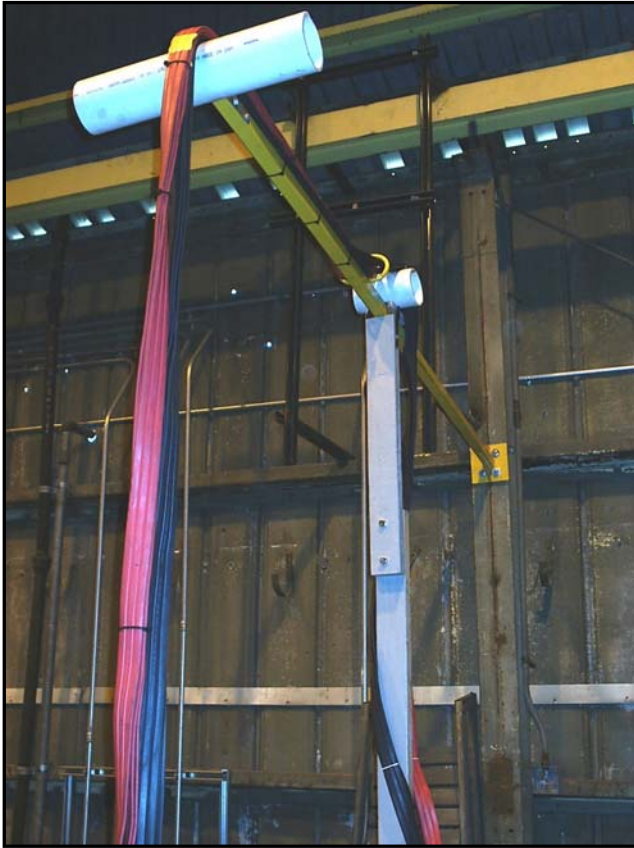
Figure 2-9. Anode and Cathode Cable Hoist System
