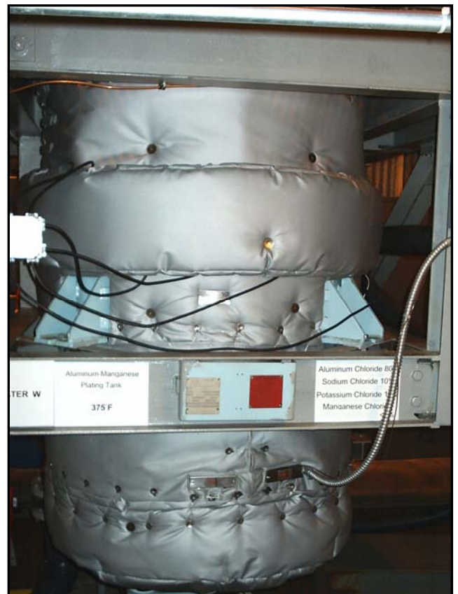
Figure 2-8. Plating Tank with Heating and Insulation Installed
