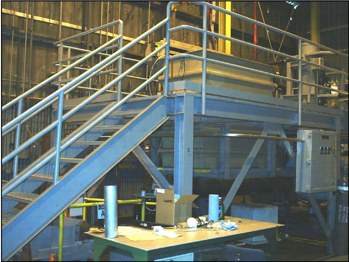
Figure 2-4. Heating System Control Panel and Chemical Add Funnel
