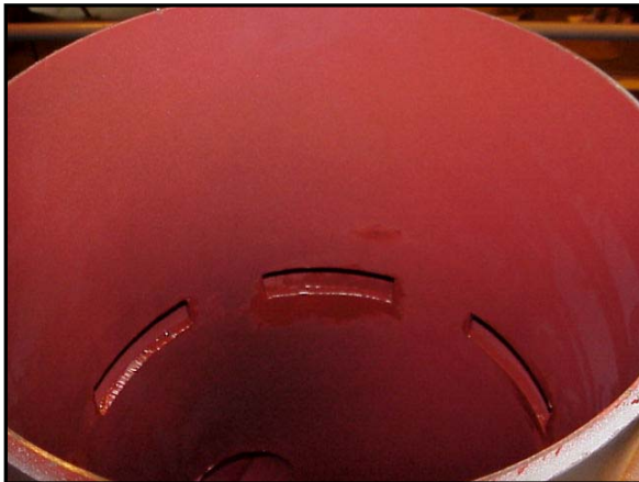
Figure 2-7. Inside Surface of Ventilation Plenum
