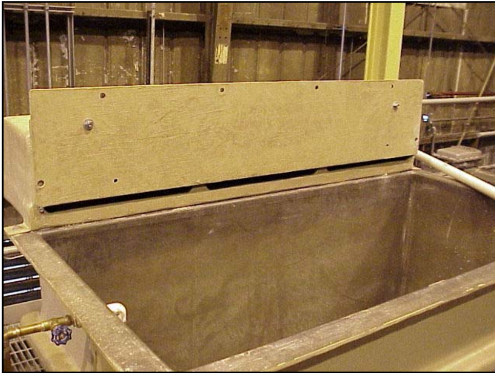
Figure 2-11. Water Rinse Tank
