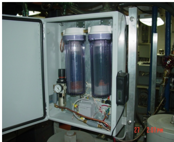
Figure 2.2 I 2 Bubble Infusion Device
