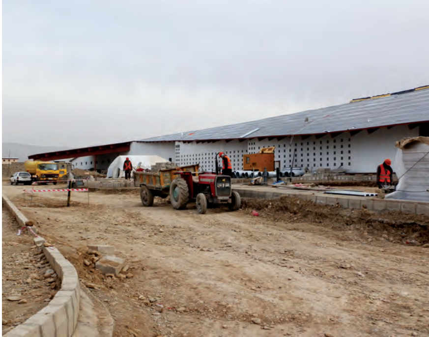
The Gardez hospital , shown here under construction, has annual operations and maintenance costs that are too high to be sustained by the Afghan government. See Inspection Report 14-6-IP and Audit Report 13-9. (SIGAR photo by Lise Pederson)
