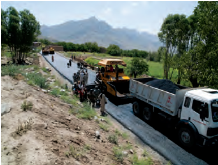
Sustaining non-security projects , like this DOD-funded road, could cost as much as 15% of Afghanistan’s GDP. See Special Project 14-72-SP. (ISAF photo)
