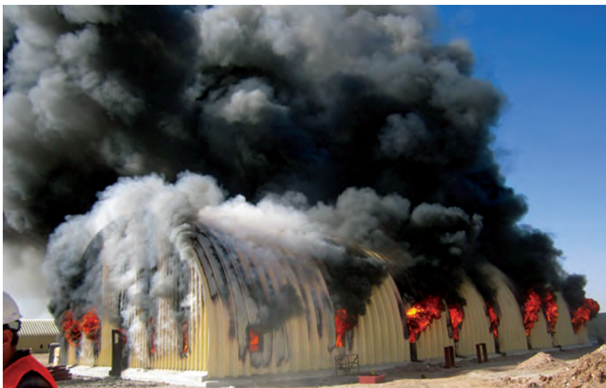
A fire at a non-code-compliant ANA classroom destroyed the structure in 30 minutes. See Special Project 14-77-SP. (USACE photo)
