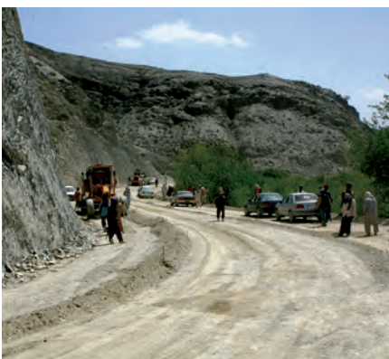
Many U.S.-funded roads , like this one from Gardez to Khowst, may not be sustainable. See Special Project 14-64-SP. (USAID photo)
