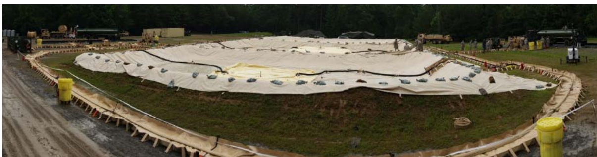
Figure 1. Fuel System Supply Point (FSSP) set up at POL Site 4 at Fort A.P. Hill during the 2014 Quartermaster Liquid Logistics Exercise (QLLEX '14).
