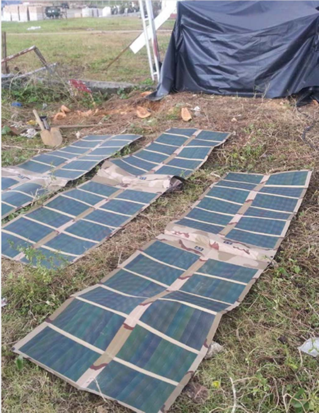
Figure 14. Solar Panels Used to Power an HFN
