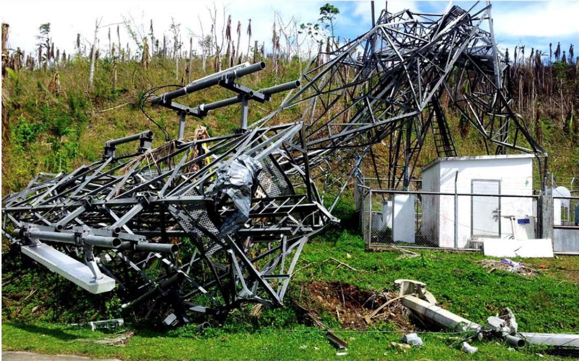
Figure 17. Destroyed Cellular Tower Near Tacloban City, Philippines.
