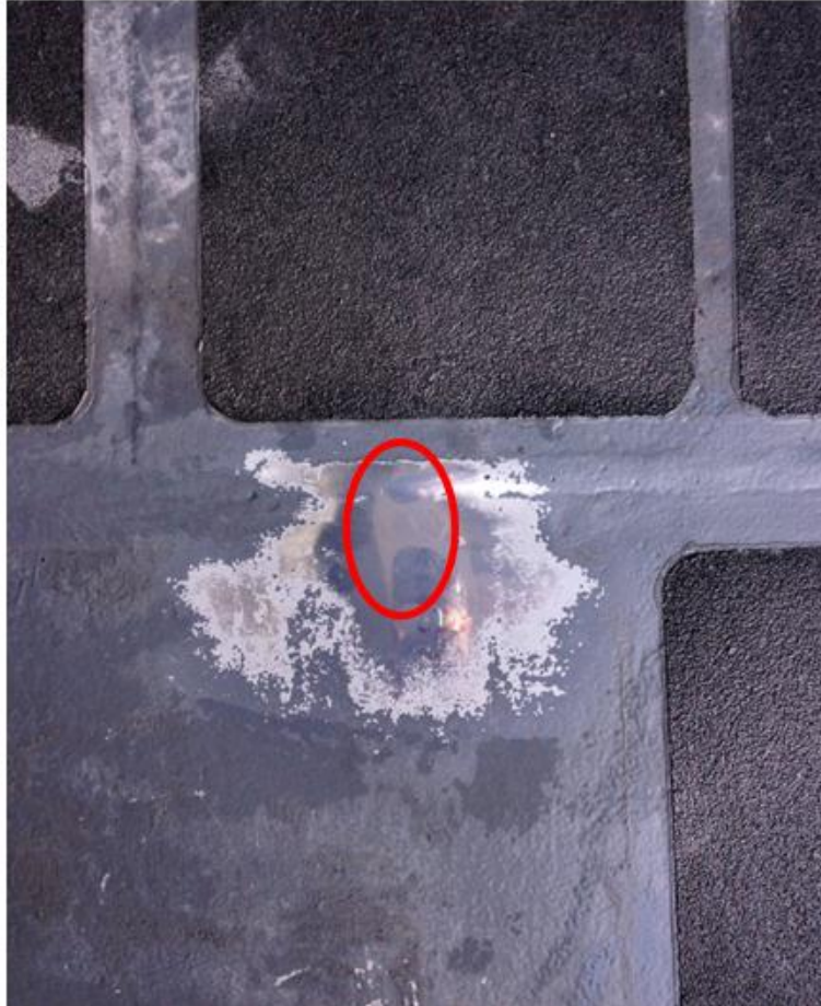
Figure 57. Position two located on the O4 deck of a U.S. Navy cruiser. The line profile was set up from the center of the weld towards the anticipated base material shown by the red oval.
