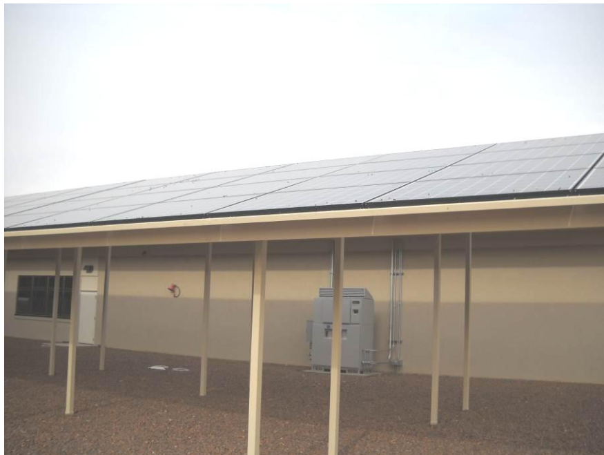
Figure 5-19 Kyocera KD210GX-LPU Solar Panel Modules
