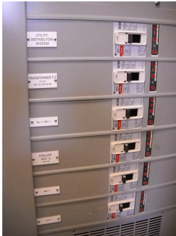
Figure 5-16 Load Breakers in Main Switchboard prior to Motor Operators Installation
