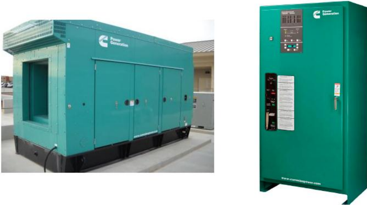
Figure 5-10 Existing Backup Generator and Automatic Transfer Switch
