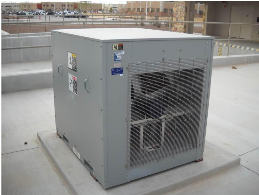
Figure 5-12 Generator Test Load Bank
