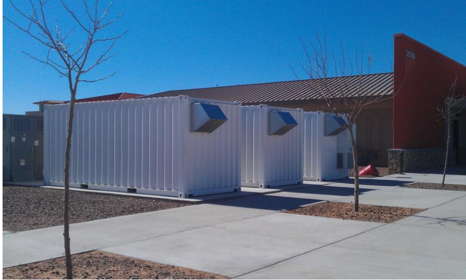
Figure 5-8 Three Energy Storage Containers at the EPDF
