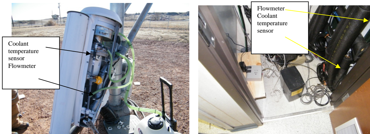
Figure 13: PowerDish and Building Flow and Temperature sensors: PowerDish (left) and Building #9246 Utility Closet (right)
