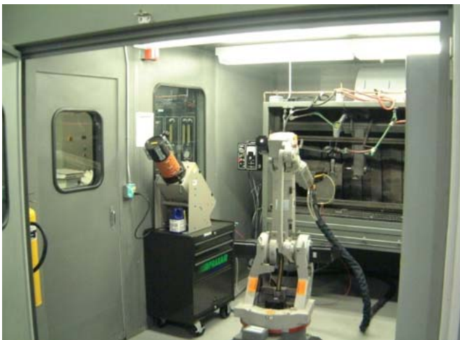
Figure 3. Inside of HVOF Spray Booth at OO-ALC.
