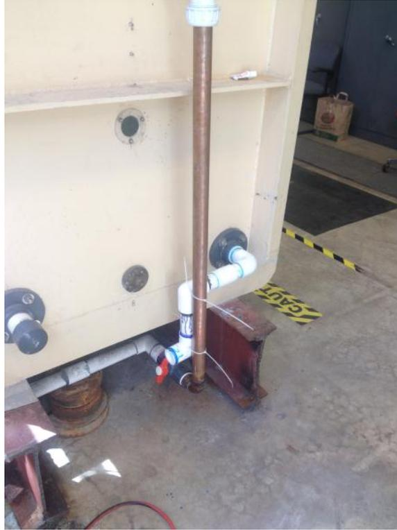
Figure 99 Tow tank fill valve at north end of the tank
