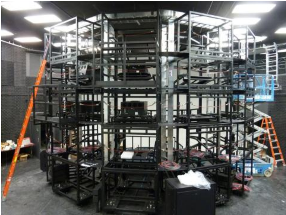
Figure 15. Completed OBVA projector structure with some projectors mounted.
