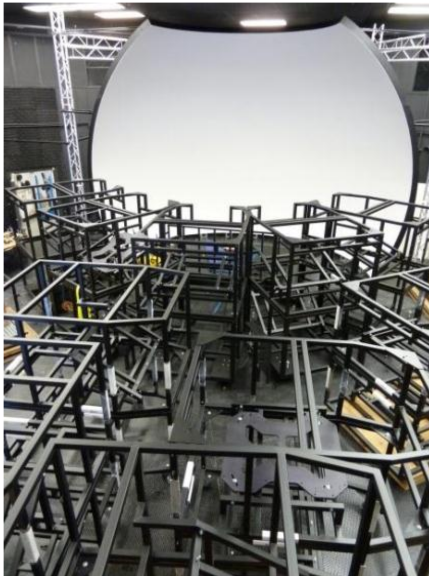
Figure 13. Initial view of OBVA projector structures.
