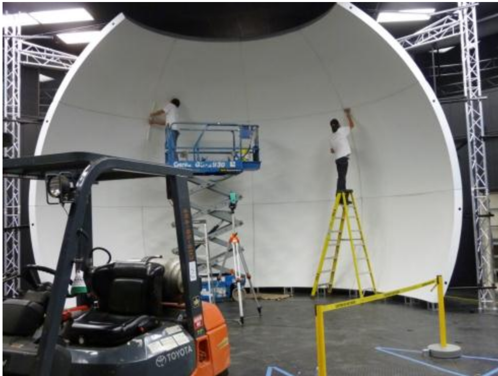
Figure 10. OBVA screen being filled with drywall compound.
