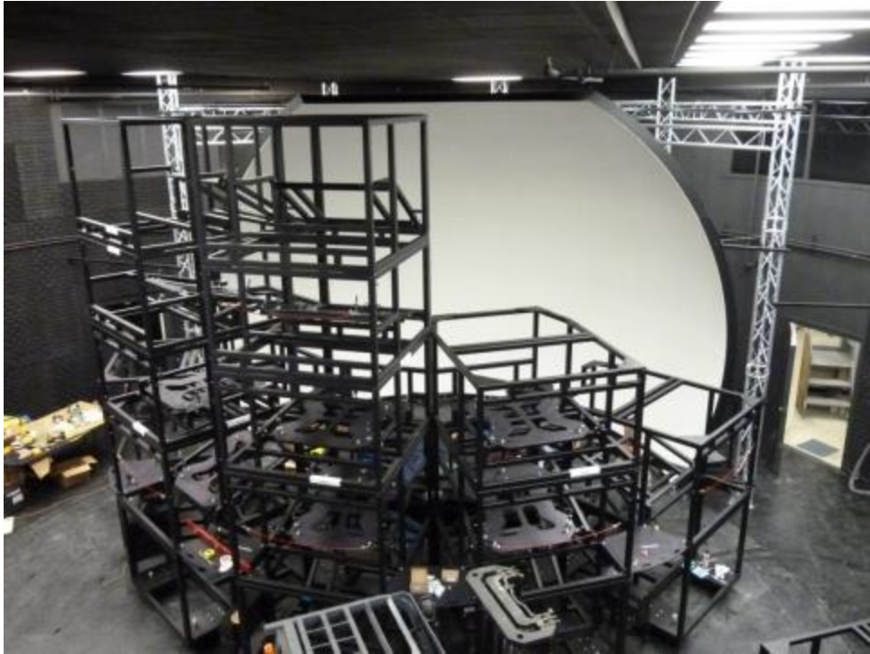
Figure 14. Partial assembly of OBVA projector structure.
