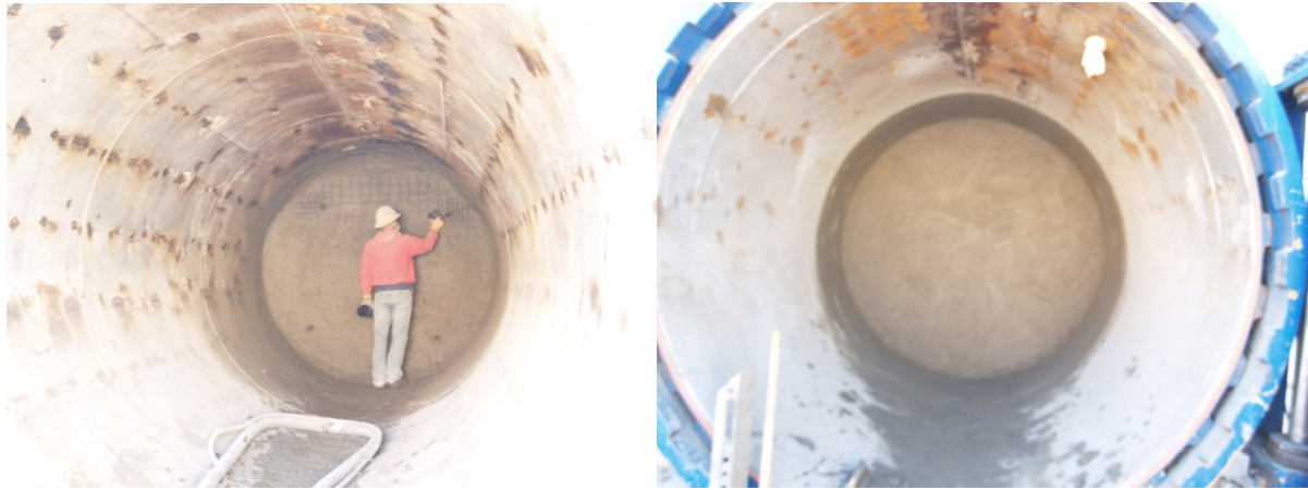
Fig. 10-6. Application of Shotcrete (left); completed concrete volume fill (right).
