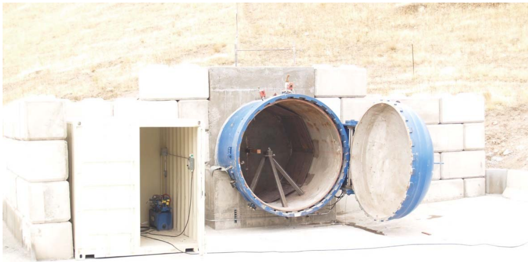
Fig. 10-10. Finished installation with hydraulics shed.
