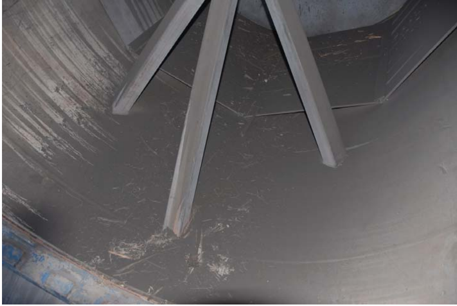
Fig. 10-15. Post-test powdery residue/ash on chamber floor.
