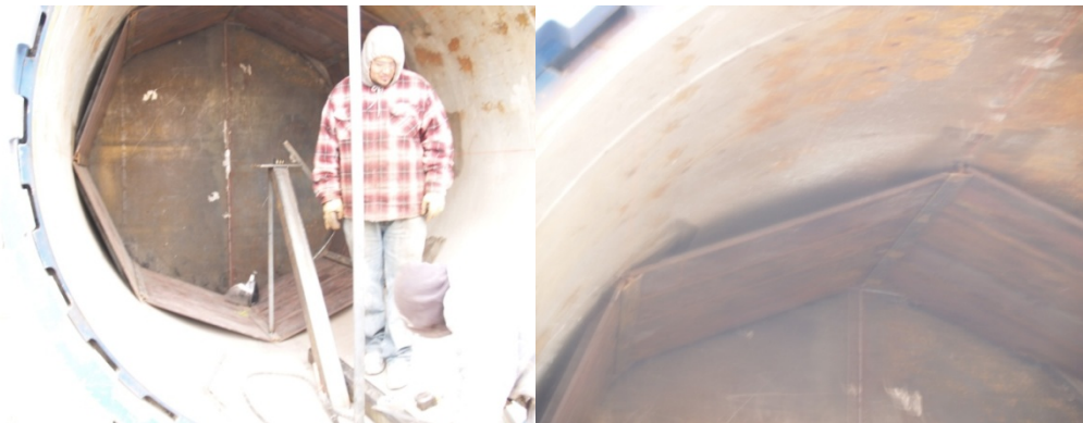
Fig. 10-7. Steel bulkhead and armor plating.
