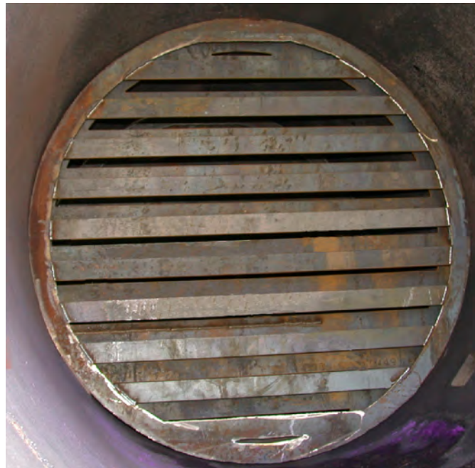
FIGURE 3-9. Baffle Detail. Two-inch stainless steel strips alternate in two layers 4 inches apart.
