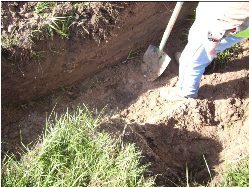
Figure 42. Cable located with the EM31 at bottom of excavation, LPV104_K. UTM Coordinate (785579.6, 3325961.8).
