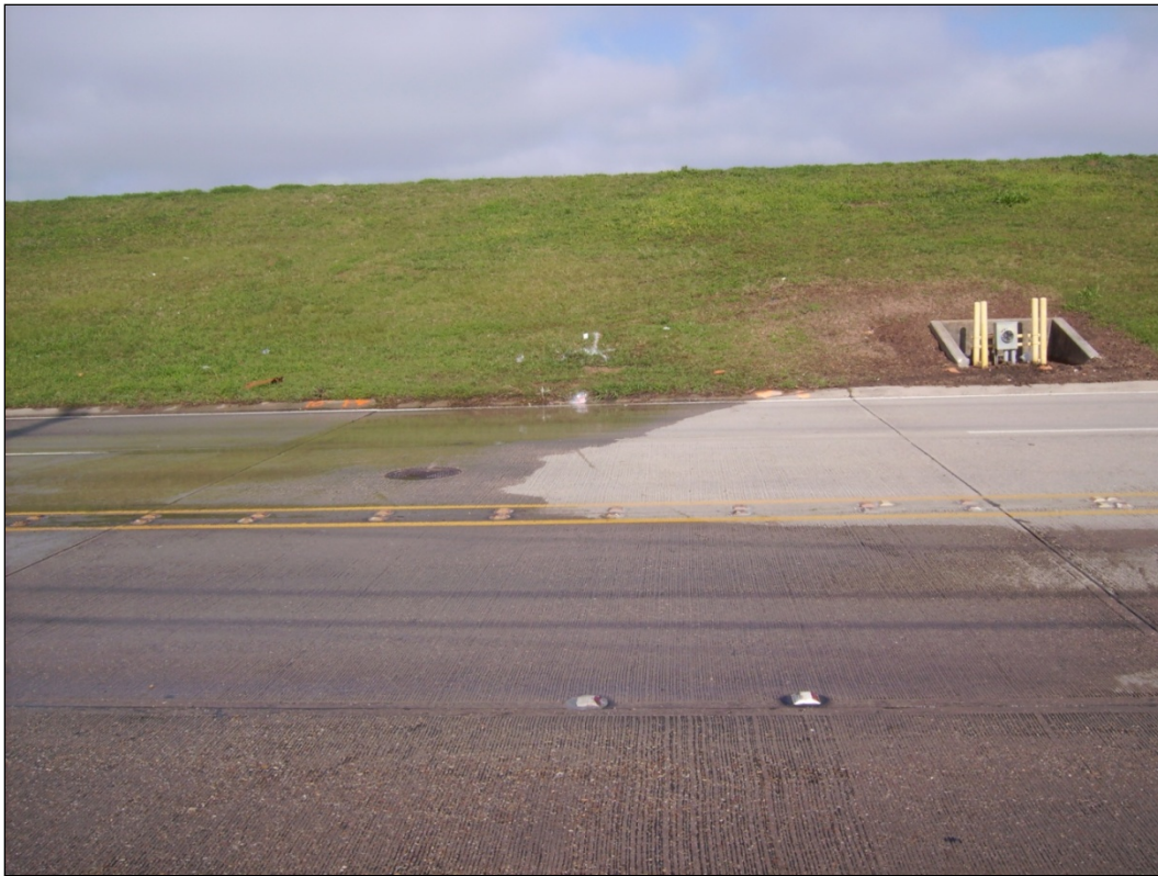
Figure 46. Seepage area, indicated by the white flag on the toe of the levee, located near the intersection of Hayne Boulevard and Pebble Drive.
