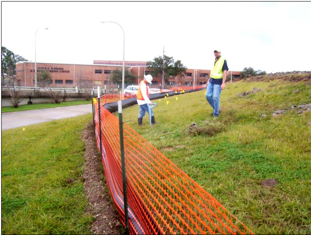
Figure 44. Radio transmitter in storm sewer being tracked on the ground surface. Yellow flags indicate storm sewer track.
