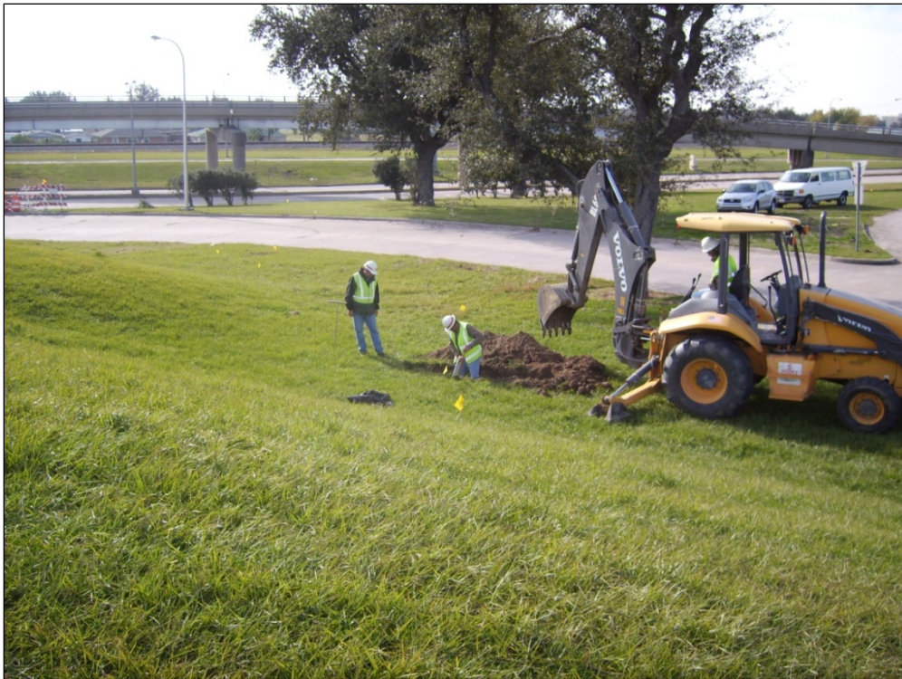
Figure 41. Excavating an EM31 anomaly marked with yellow flags, LPV104_K. UTM Coordinate (785579.6, 3325961.8).
