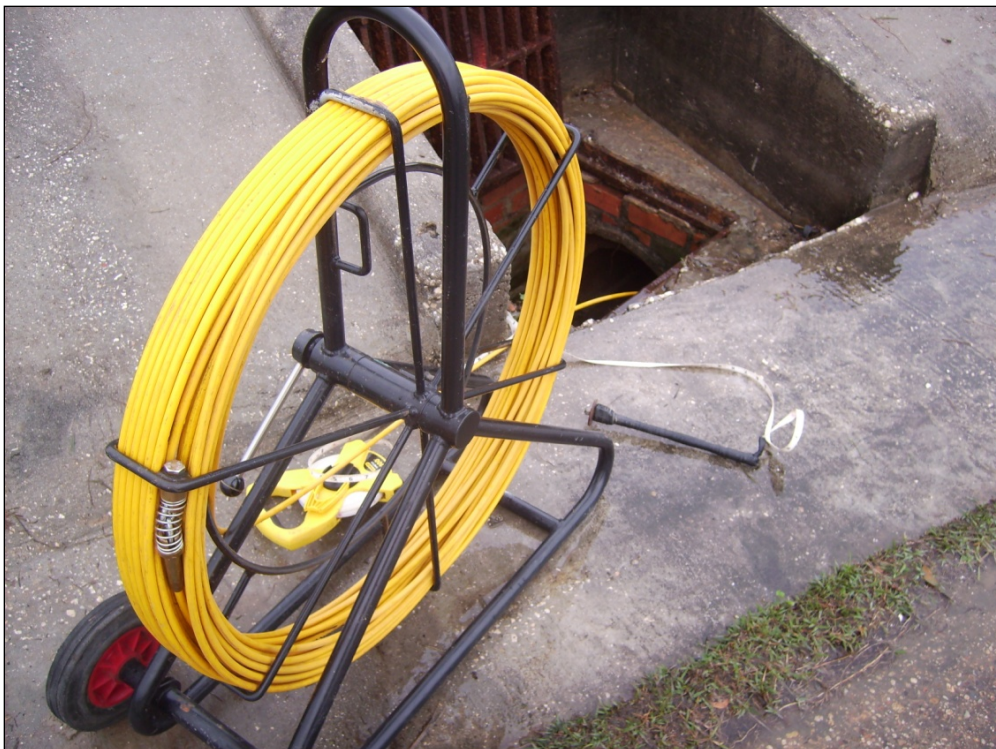
Figure 43. Radio transmitter placed in storm sewer, UTM coordinates (785524.6, 3325885.6), LPV104_K.
