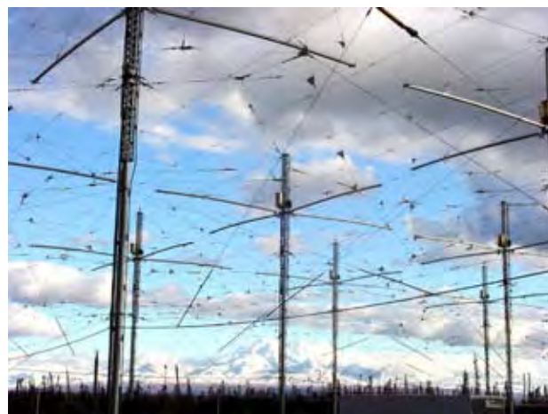
Antenna Farm in Gakona, Alaska (U.S. Air Force photo)
