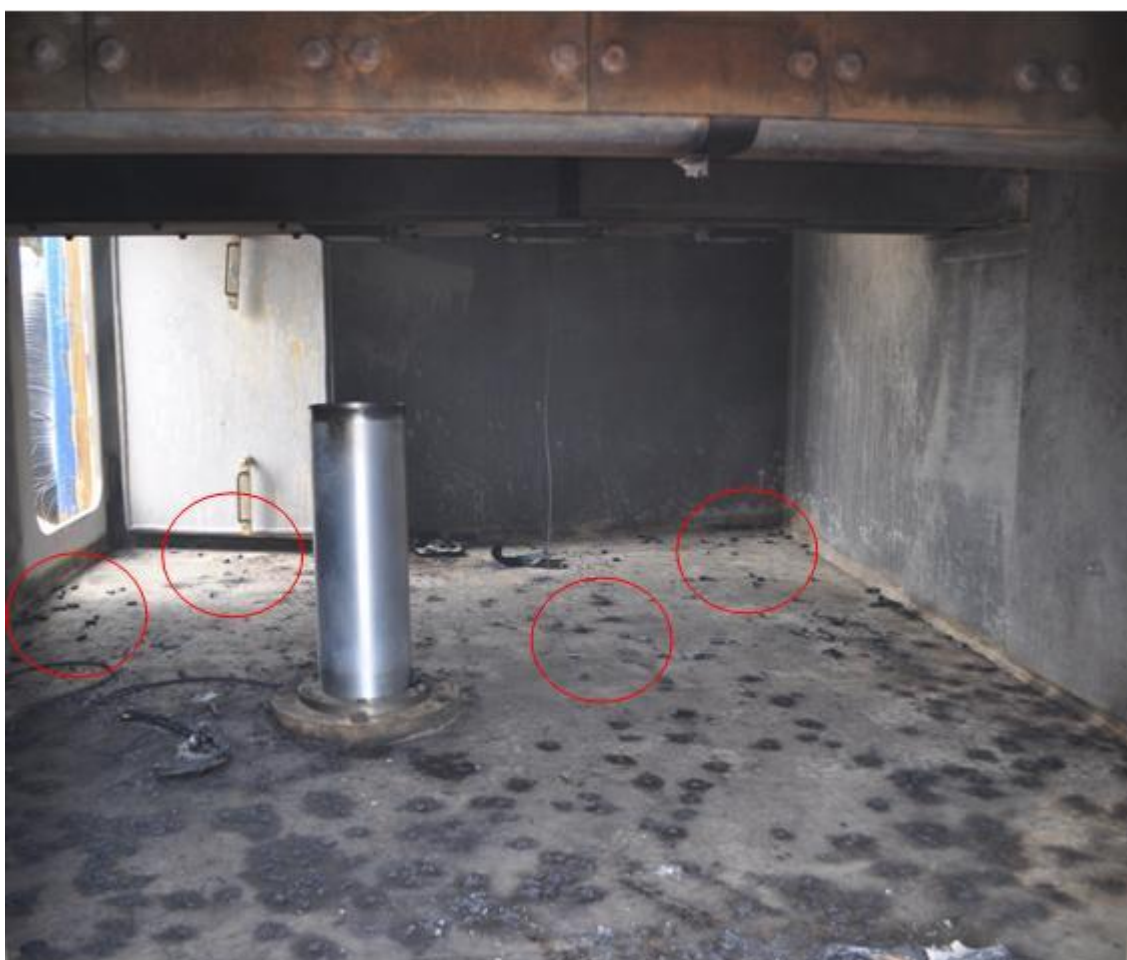
Figure 11: Burn marks suggesting a reduced dispersion of combustion zones in the absence of a storage tube end-cap. Locations of unburnt propellant grains are circled.
