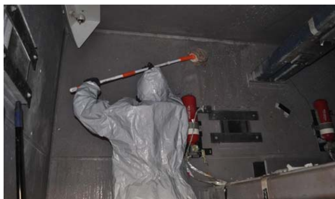
Figure 41: Mopping down of the trials structure with calcium carbonate/water emulsion after preliminary dusting with calcium carbonate
