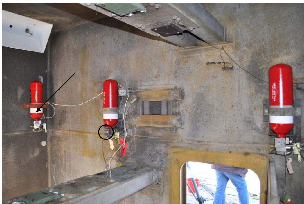
Figure 9: Extinguisher configuration on one side of the trials structure for the combined water and gaseous suppressant experiment (Experiment 13)
