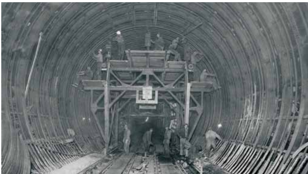
Tunnel # 1 under construction in 1936. Workers place steel reinforcing for sidewall and arch of the tunnel. This tunnel would be steel lined, unlike the other three tunnels, in preparation of a powerhouse to be built at the outlet of the tunnel.
