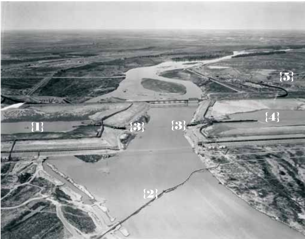
Fort Peck Dam in 1936 showing the west and east core pools with the river open in the center.
