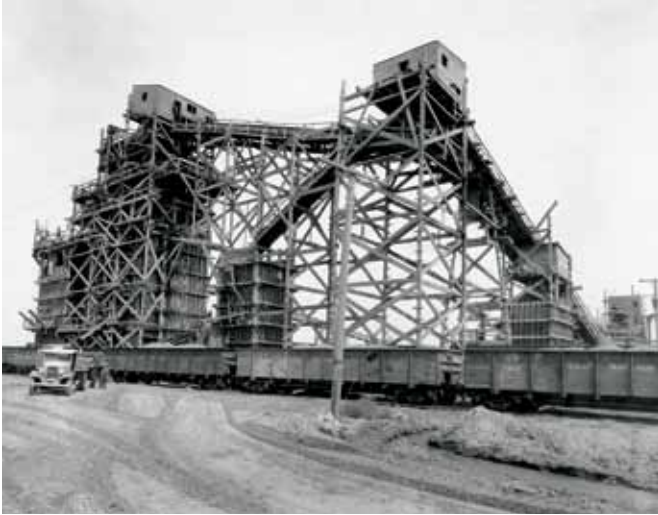
Above: The huge gravel plant was capable of producing 100 train carloads of screened and washed gravel each day.
