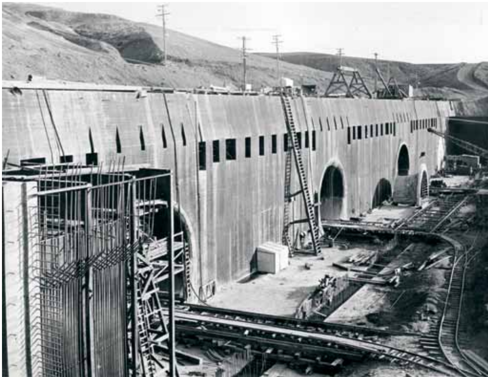
The tunnel intakes under construction in 1936. These intakes are now submerged under 200 feet of water at the bottom of Fort Peck Lake.
