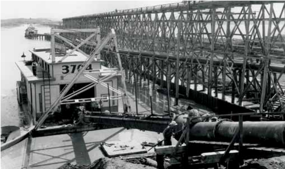
Workers connecting the newly relocated pump boat 3704 back into the pipeline. The pump boat is in the core pool, on what is now the top of the dam. Timber cut in the area that would become the reservoir was used to build the support trestles for the 28-inch pipeline.
