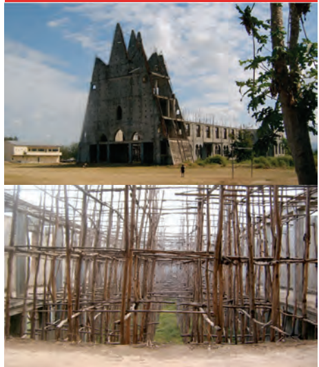
The Suai Cathedral was under construction at the time of the 1999 massacre and has not been touched since.
