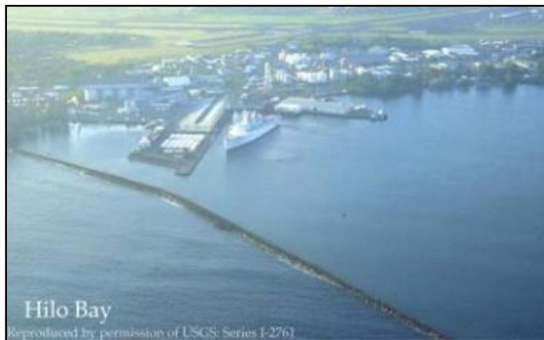
Figure 25. Hilo Harbor breakwater and berthing areas, Island of Hawaii. The Hilo Small Boat Harbor is also visible in the upper left portion of the photograph (uncaptioned figure of UH CGG 2012; by permission).
