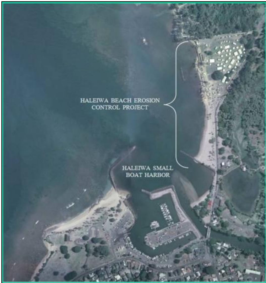
Figure 11. Google image (30 July 2006)–Haleiwa Small Boat Harbor and the Haleiwa Shore Protection Project.
