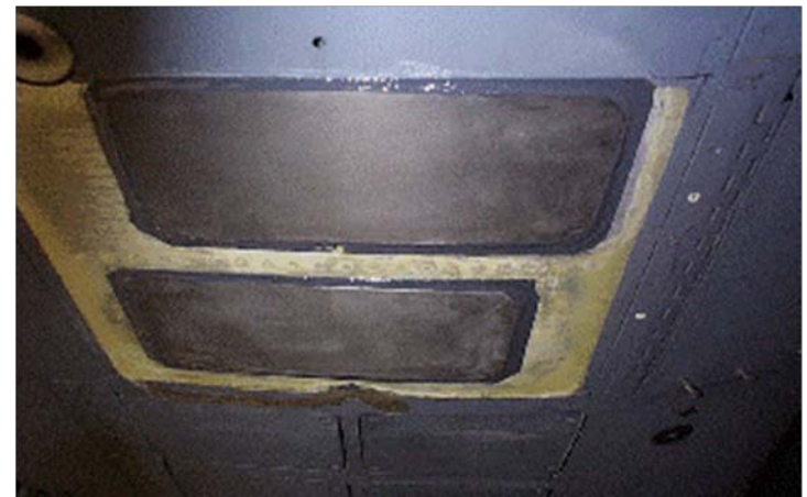
Composite Patch Repair
