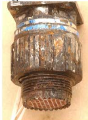
Figure 6.1.6 Corrosion resistant stainless steel after 336 hours in SO 2 -salt fog
