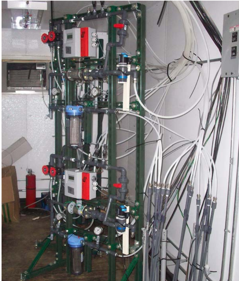
Figure 5-19. Photograph of Amendment Injection Rack
