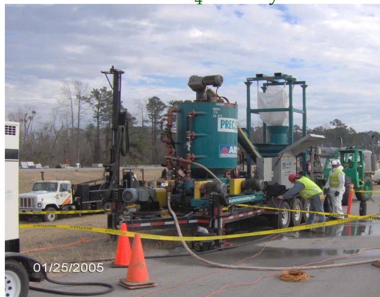
automatic \text{KMnO}_4 feed system
