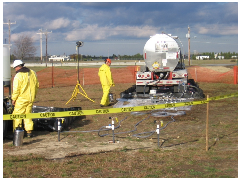
automatic \text{KMnO}_4 feed system
