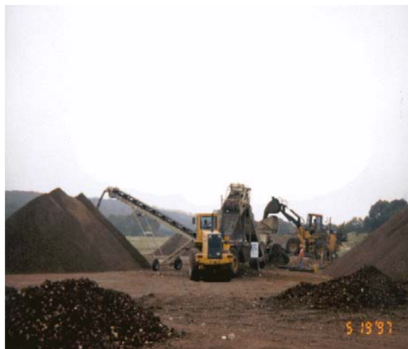
Figure 6. Sieving to Remove UXO and Large Metal Debris.
