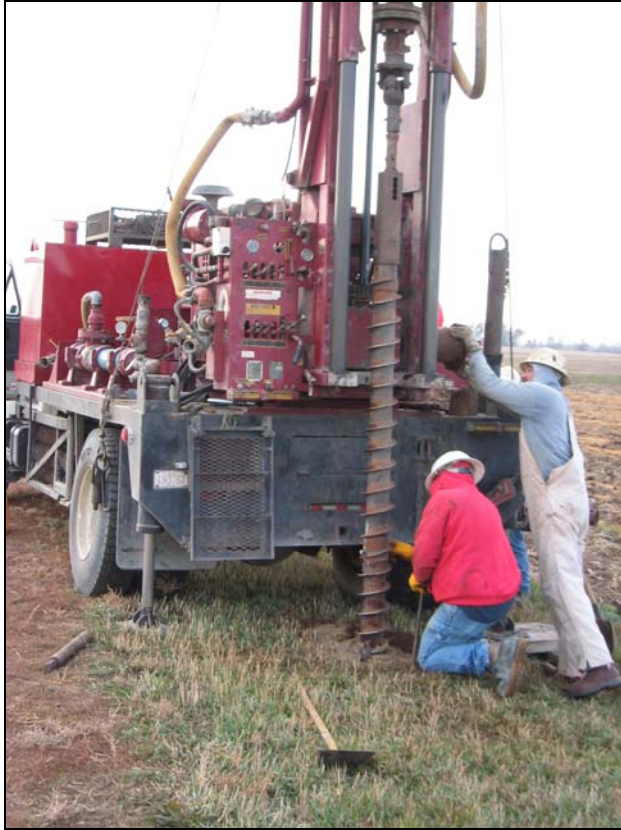
Figure 9. Installation of MW-01
