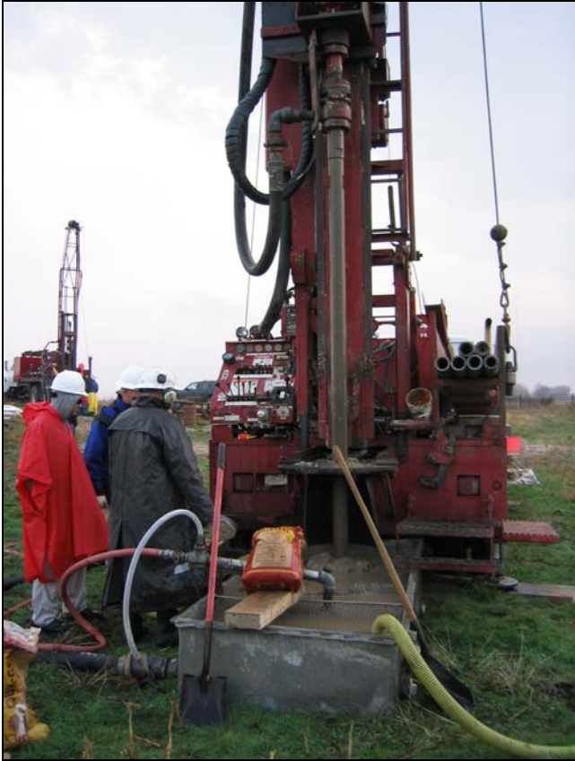
Figure 6. Installing extraction well (EW-01)
