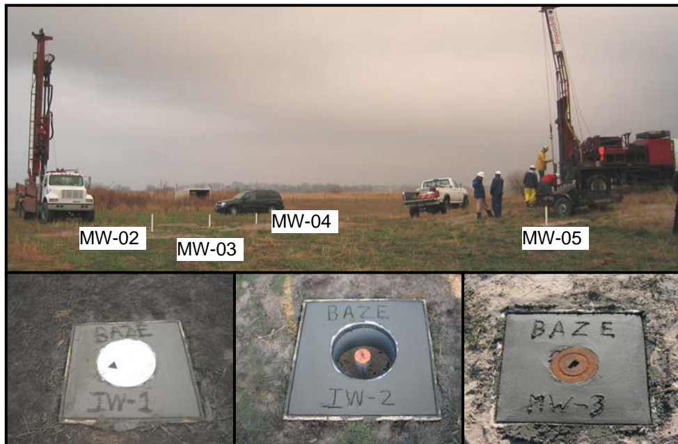
Figure 10. Installation of wells (above) and final product (below).
