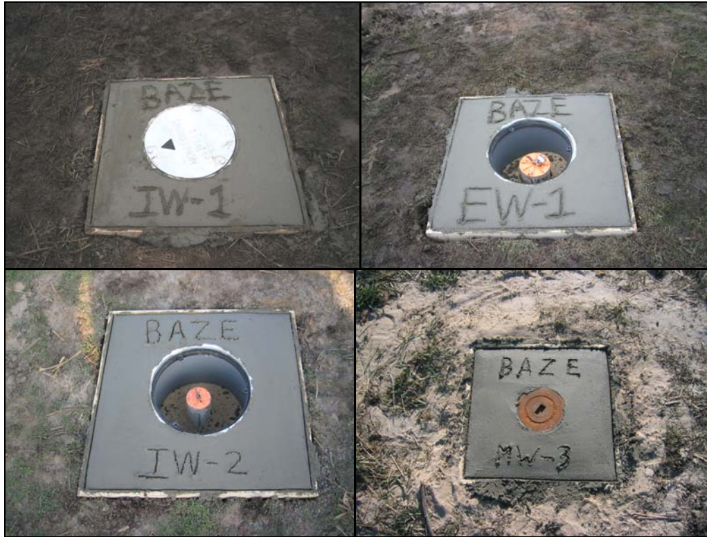
Figure 7. Photo of injection wells 1 & 2, extraction well 1, and monitoring well 3
