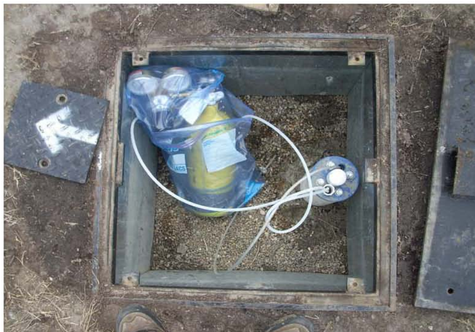
Compressed Air Cylinder
