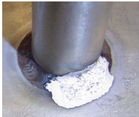
Figure 30 - Thermionically Cleaned Tube-Sheet Joint
