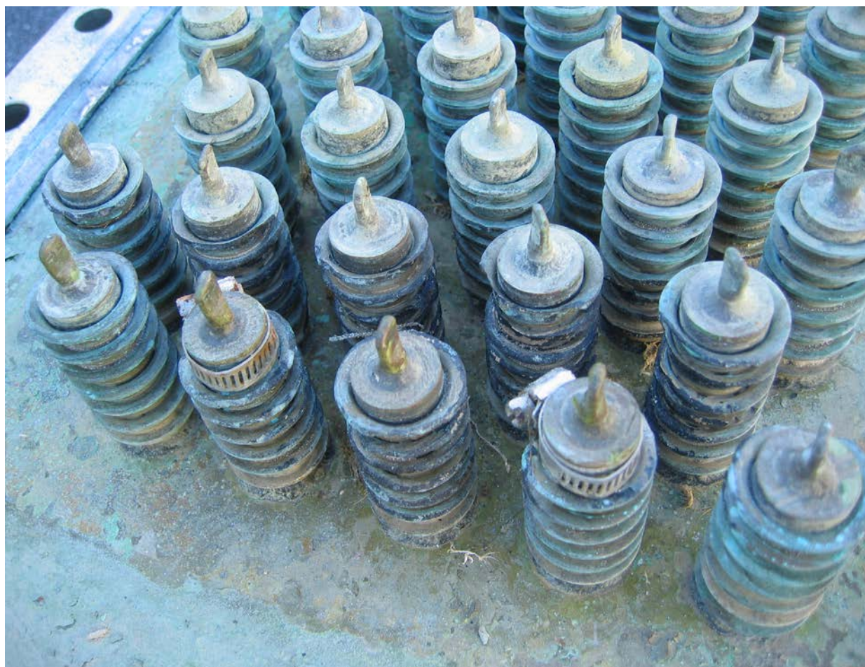
Figure 1 shows impingement damage to the heat pipes near the water inlet.
