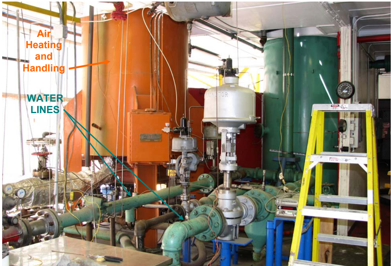
Figure 25 Test Facility Air and Water Equipment Inlet Side
