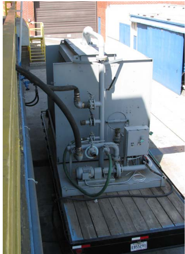
Figure 27 Heat Exchanger (outside)
