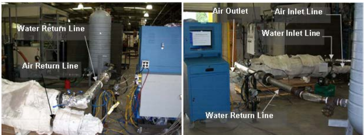
Figure 7- 3 HP-BAC Test Setup at Stork East-West Technology Corp.
