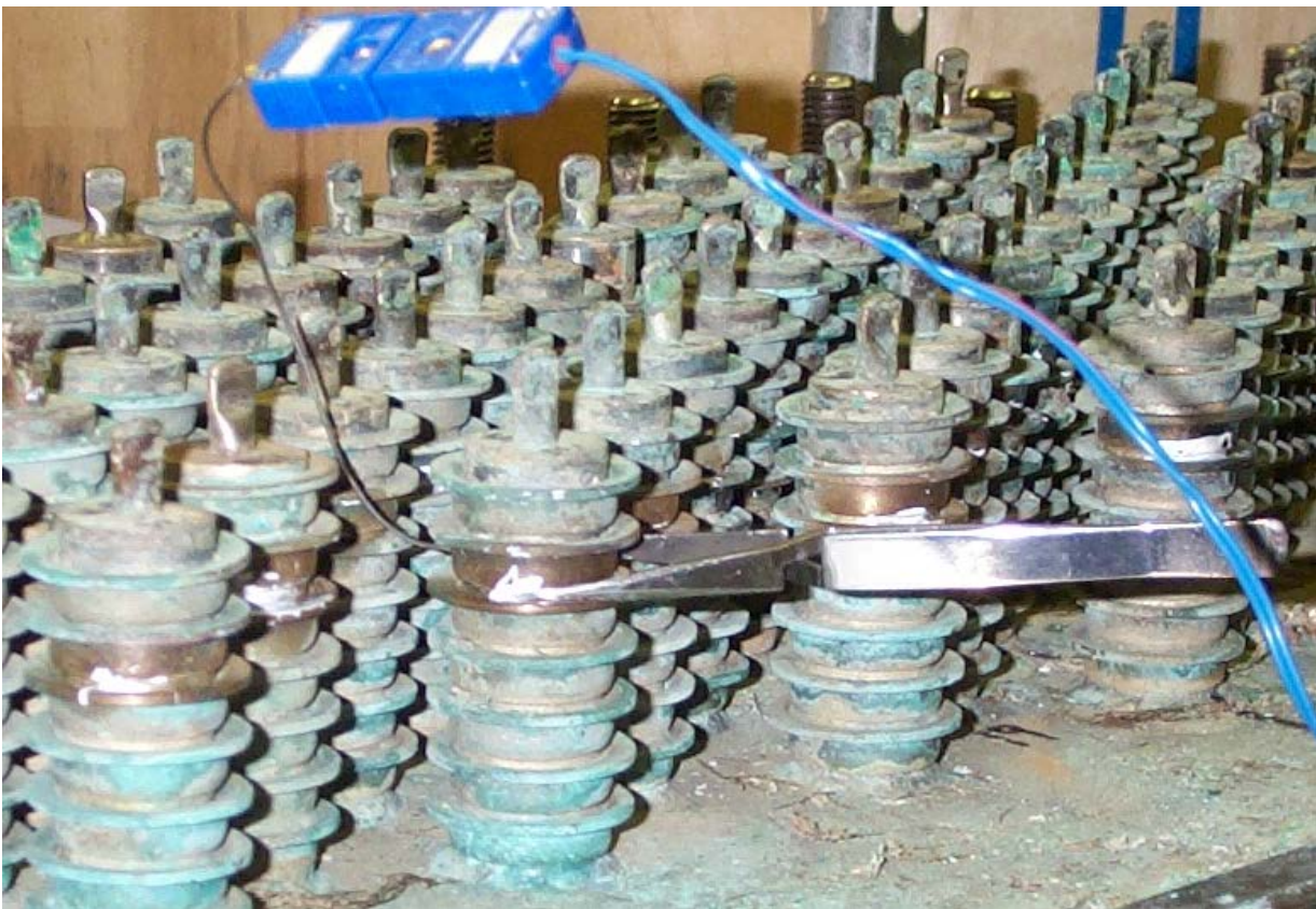
Figure 3 – Upper end of a heat pipe during a performance verification test.
