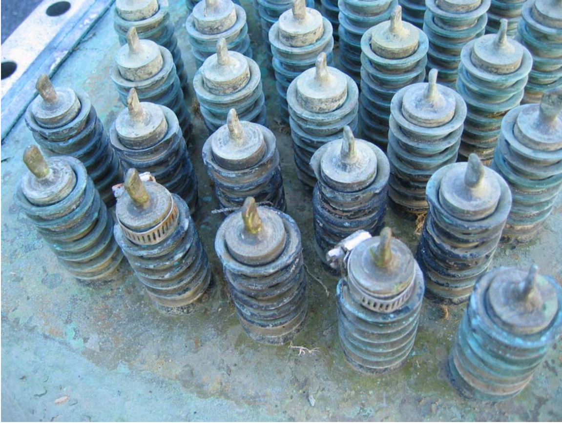
Figure 1 Impingement Damage to the Heat Pipes near the Water Inlet.
