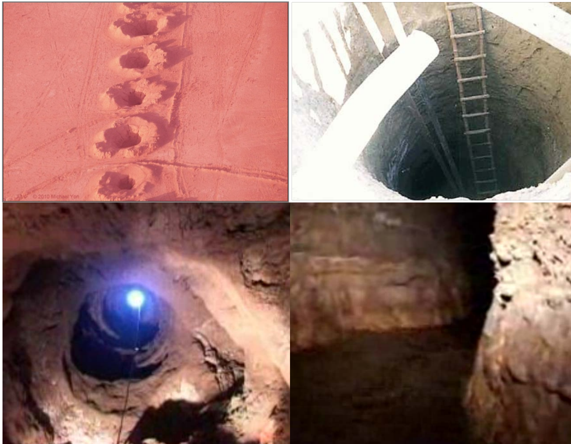
Figure 4.6. (UL) low-altitude view of chahs in southern Afghanistan, scale provided by vehicle tracks (image courtesy of Michael Yon); (UR) access shaft of a chah (USAID); (LL) view up a chah shaft during maintenance-rope attached to haul bucket (Iranian Public Television); (LR) interior of an operating karez conduit (Iranian Public Television).
