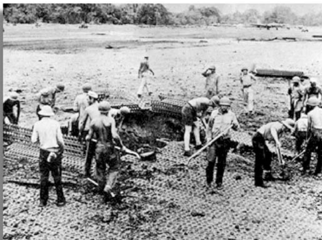
Repairing the Marston Matting. Day and night, Japanese planes attacked Henderson Field. Here US Navy, Marine, and Army men band together to repair the bomb-wrecked steel-matted runway ( http://www.daveswarbirds.com/cactus/cactus.htm ).
