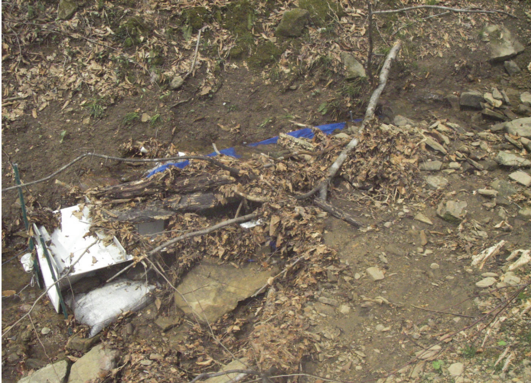
Figure 5.3.3. Evidence of debris flow at Site 3.
