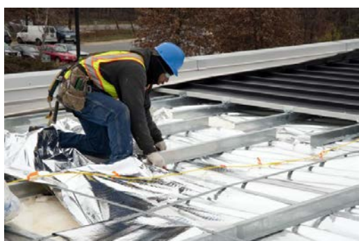
Figure 19. Army Research Lab low slope air heating roof.
