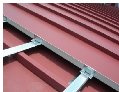
Figure 20. Metal over metal solar re-roof.
