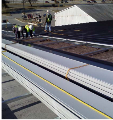
Figure 1. Solar air heating roof installation.
