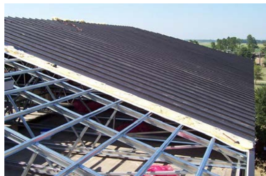
Figure 18. Sloped built-up roof example.
