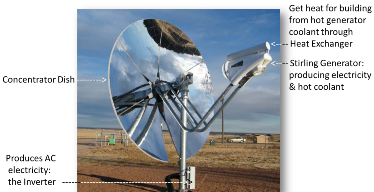
Figure 3. PowerDish CHP (heat exchanger mounted on Infinia PowerDish).
