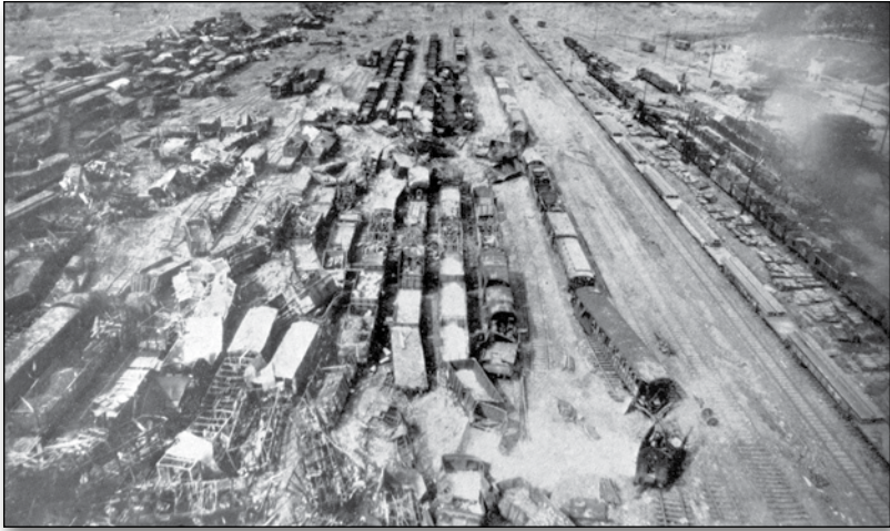
The Fulda rail yard was an important transshipment point in the German rail system that was virtually destroyed by Eighth Air Force bombers.
