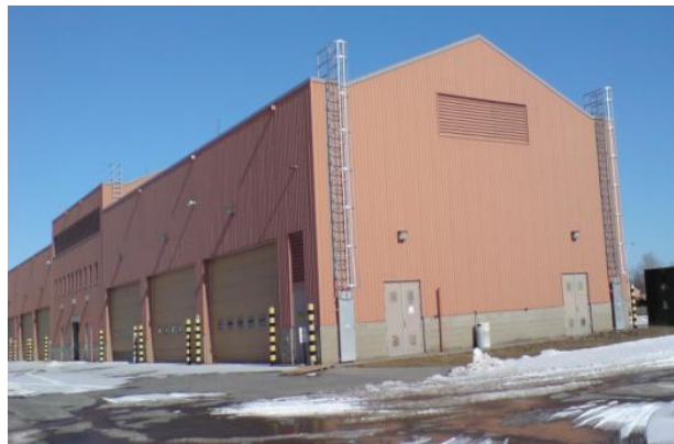
Figure 25. Tactical Equipment Maintenance Facility at Fort Drum, NY.
