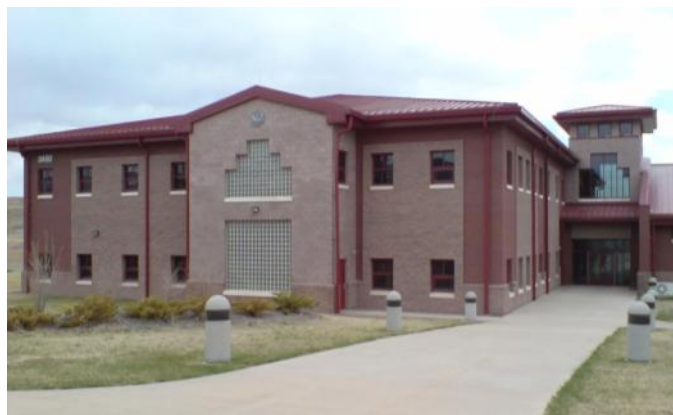
Figure 30. Army Reserve Center Bldg at Fort Carson, CO.
