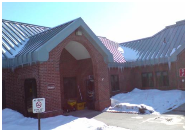
Figure 29. Child Development Center Bldg at Fort Drum, NY.
