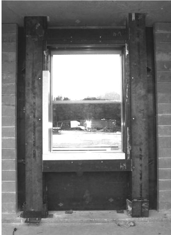
Figure 39. Bracing flanks the window and transfers loads to the floor and ceiling. Photo credit: USACE Omaha District Protective Design Center. Used with permission.
