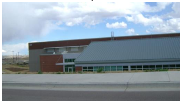
Figure 26. Company Operation Facility, Administration Office Building at Fort Carson, CO.
