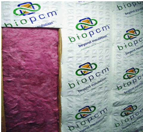
BioPCM blanket installed over insulation.
