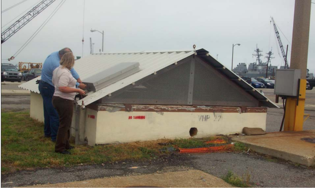
Figure 4. Photograph of a valve pit along the pipeline. The gray access hatch for human entry is located on the corrugated roof and the “access box” was mounted on the concrete wall for easy electrical connections to the transducers inside the pit.
