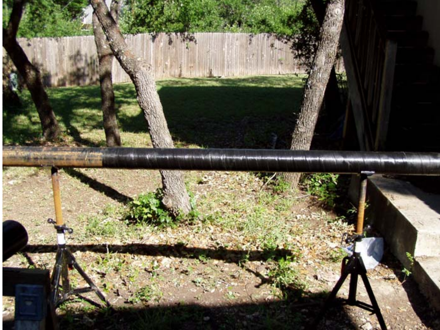
Figure 13. Pipe with wrap coating on a stand ready for ultrasonic guided wave testing.
