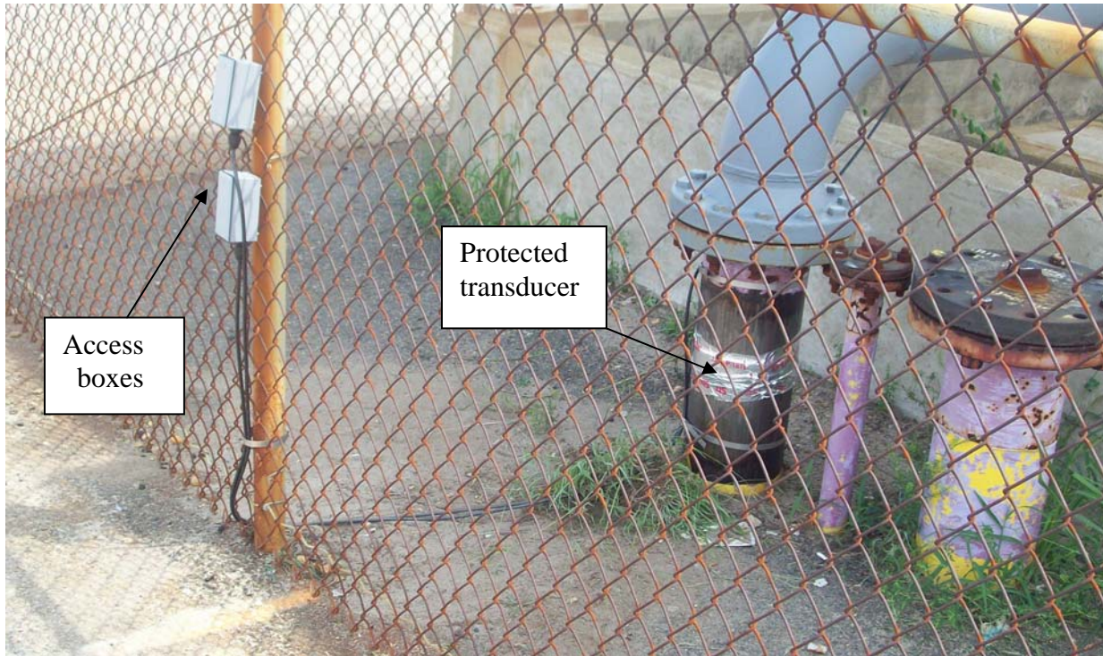
Figure 15. Access boxes for signal monitoring outside of restricted areas around VP5.
