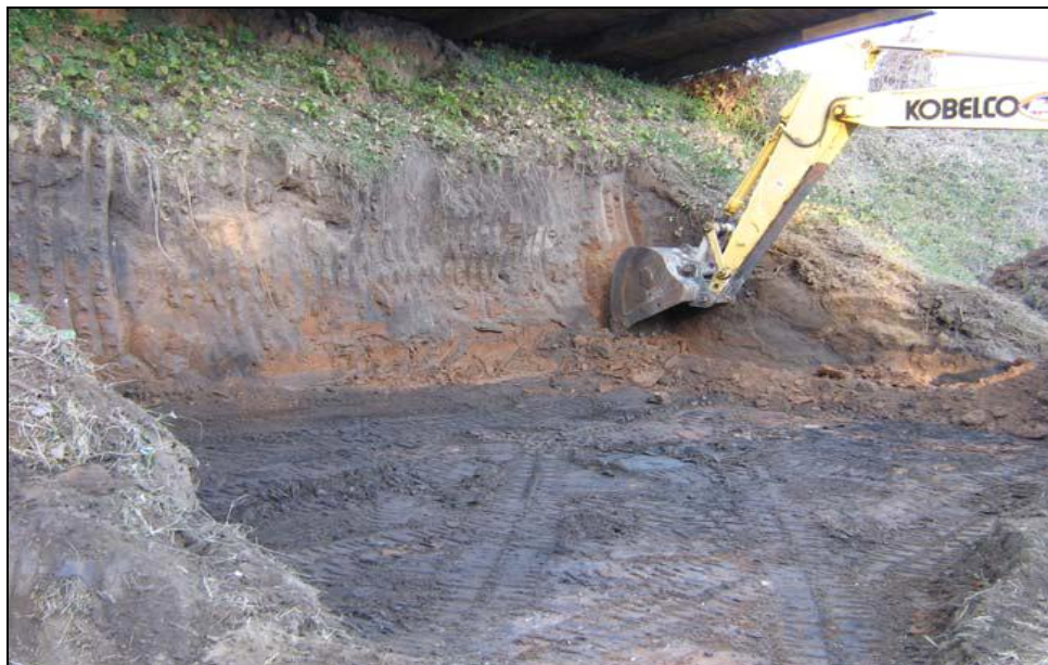
Figure 11. Removal of the old impact berm composed of local soil from under the newly constructed protective eyebrow.
