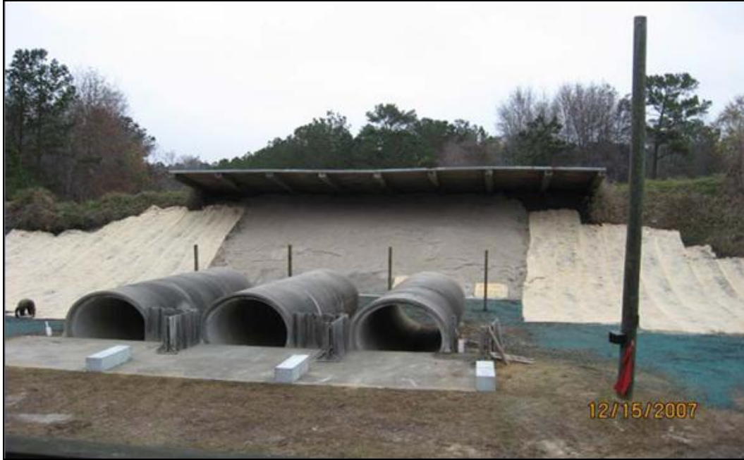
Figure 14. The completed impact berm enclosing the three experimental treatment lysimeters on the M-60 range, CAFB.
