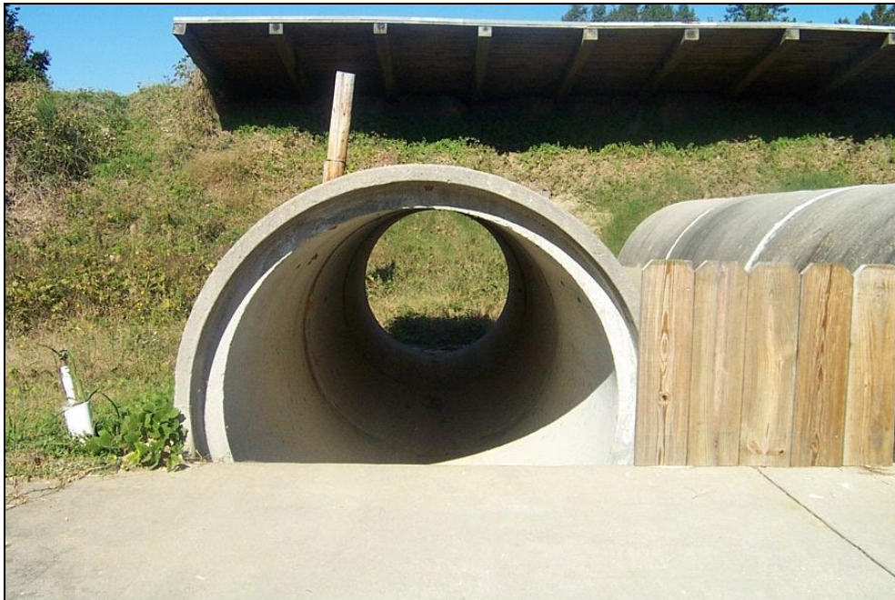
Figure 5. Preconstruction close up view through the pipe that forms the firing line looking toward the berm.
