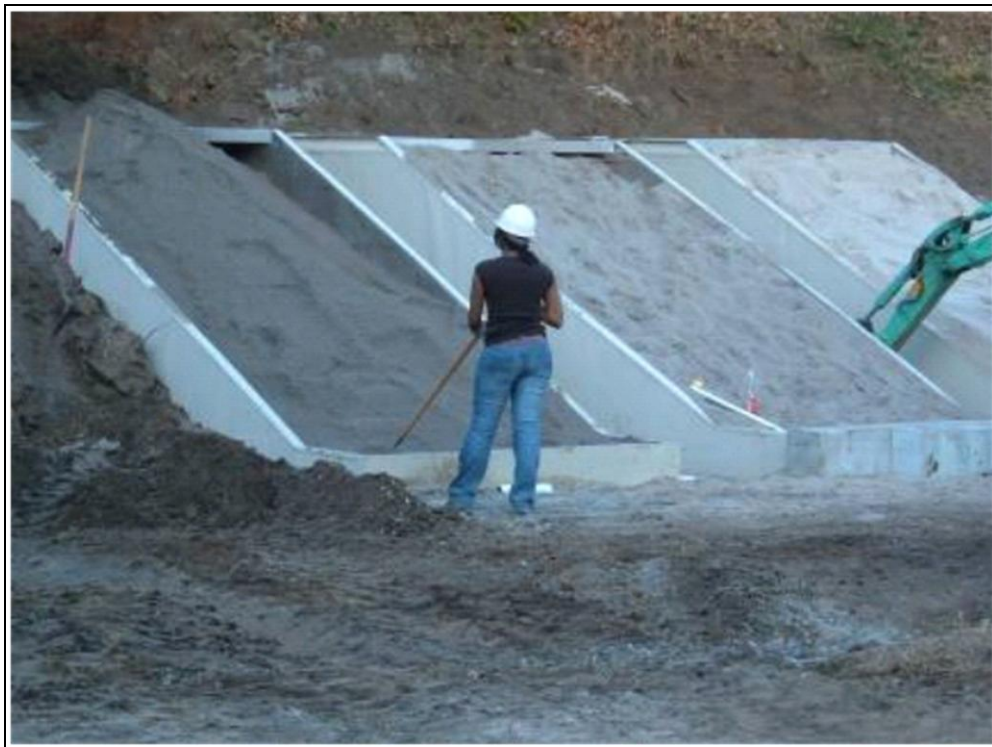
Figure 13. Placement of the amended ballistic sand in the lysimeters.
