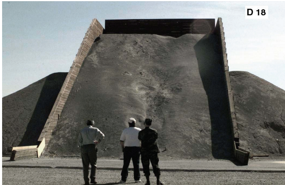
Figure 1-2. Typical catchbox at an Army test range (from Larson et al. 2009).
