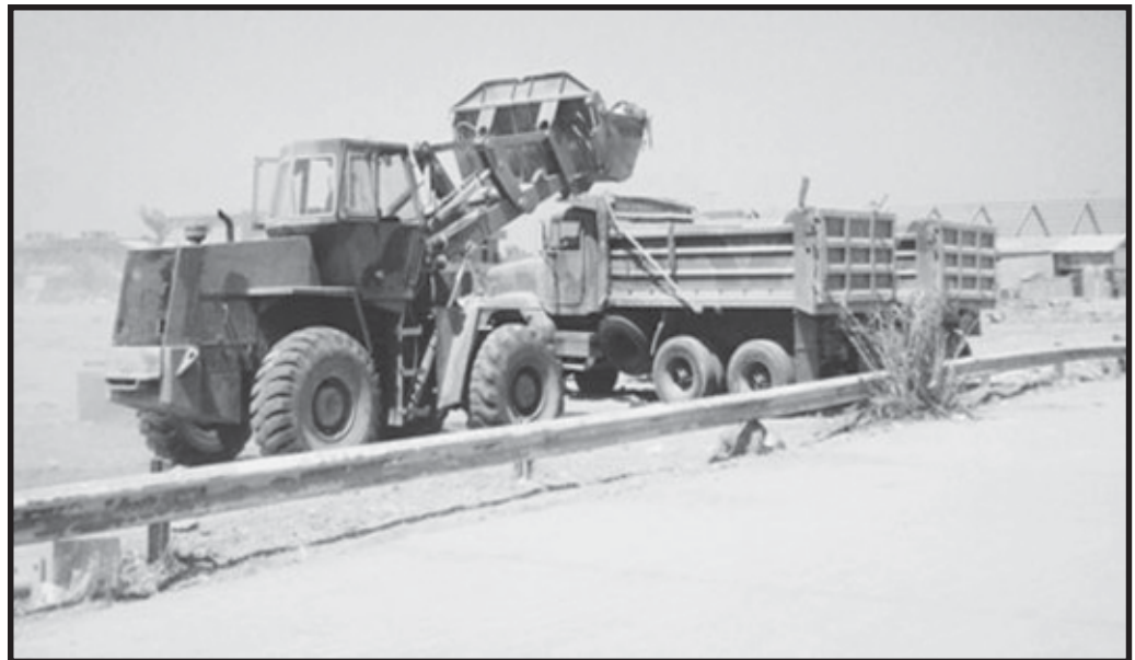
Engineer equipment was critical in the cleanup of this refugee camp.
