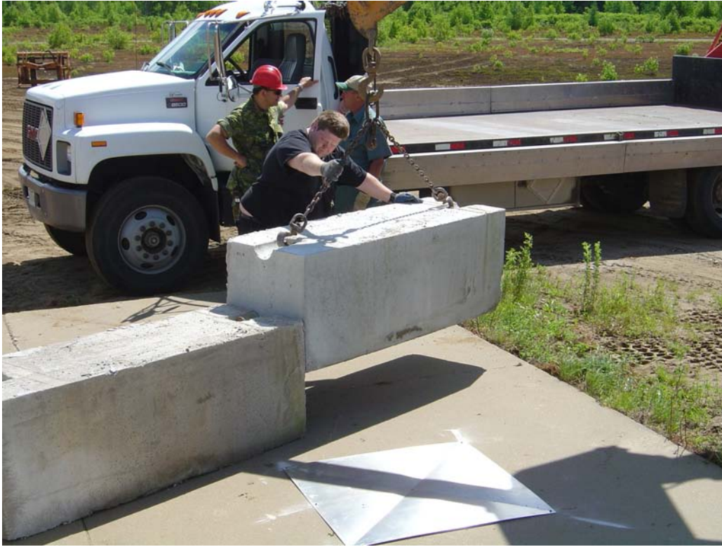
Figure 6: Installation of the concrete wall.
