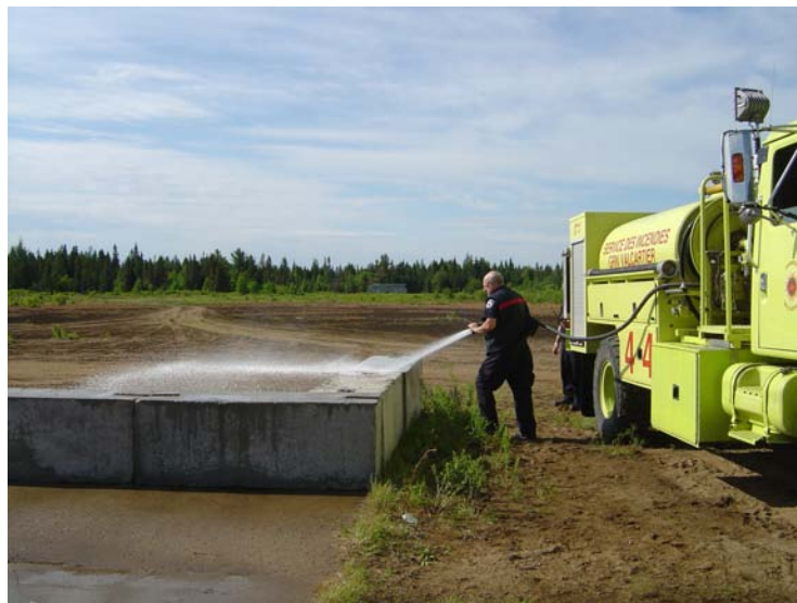
Figure 9: Washing of the concrete surfaces.
