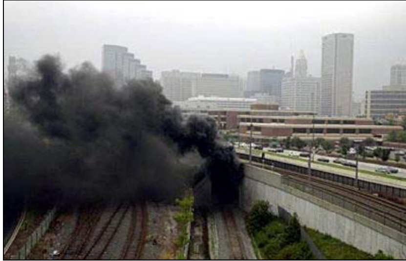
Figure 3. Smoke Billows from Howard Street Tunnel’s South Portal, with the Baltimore City Skyline in the Background 55
