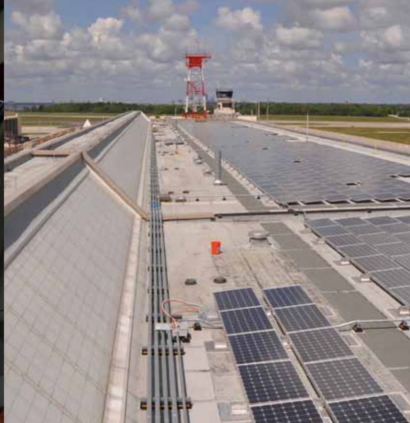
Some of the 2,534 solar photovoltaic (PV) panels installed on the roof of Naval Air Station Jacksonville's Hangar 1122 to help reduce the building's conventional energy usage and promote environmental sustainability.
