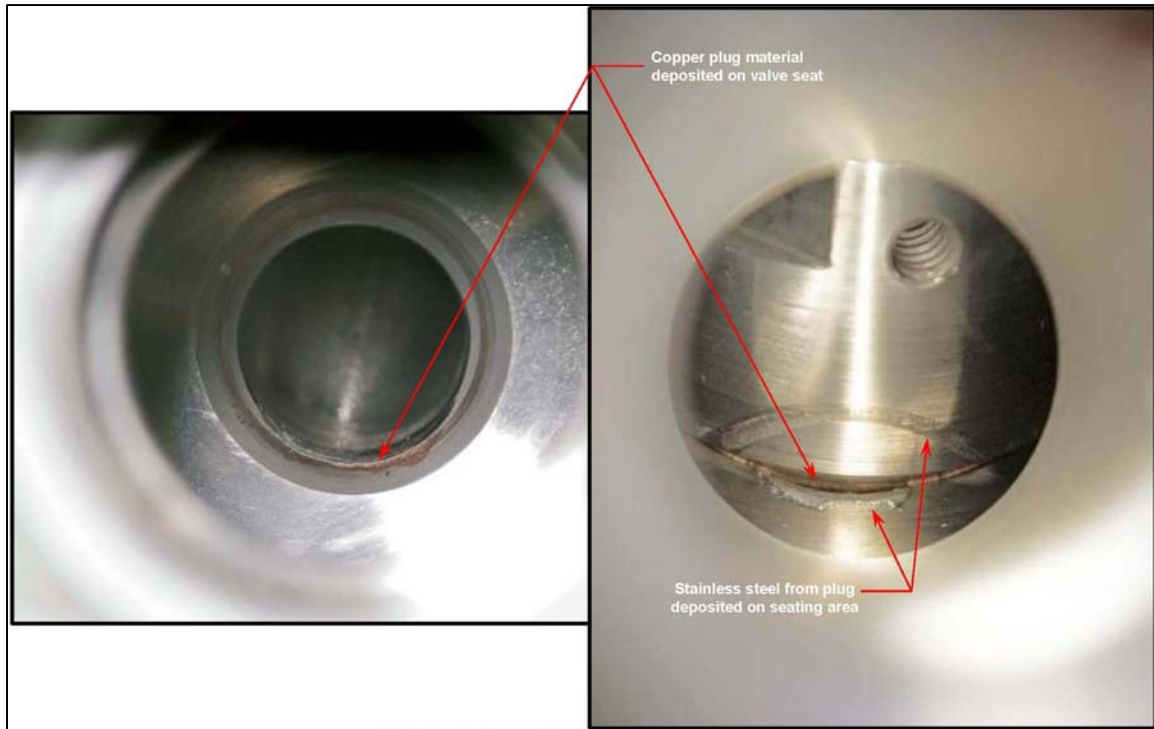
Figure 5. What you are looking at is the seating area of the valve body. Note that stainless steel in the seating area has been scrapped so hard that the plug contact area has rolled over where the plug contacted. Also, you can see where we found copper from the valve plug deposited on the valve seat.
