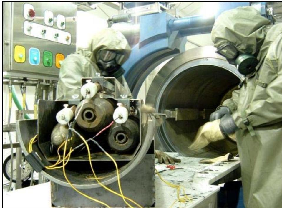
Figure 1. Illustrations of the EDS. Upper panel is the overall system and lower panel is 3 munitions being readied for detonation. (Photographs courtesy of U.S. Army<sup>10</sup>)
