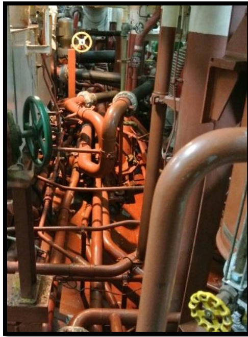
Figure 1 - Complex, space constrained piping
