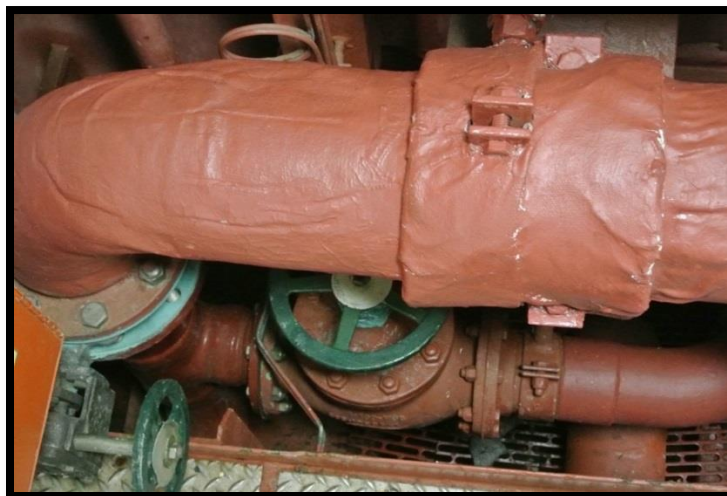
Figure 2 - Pipe lagging
