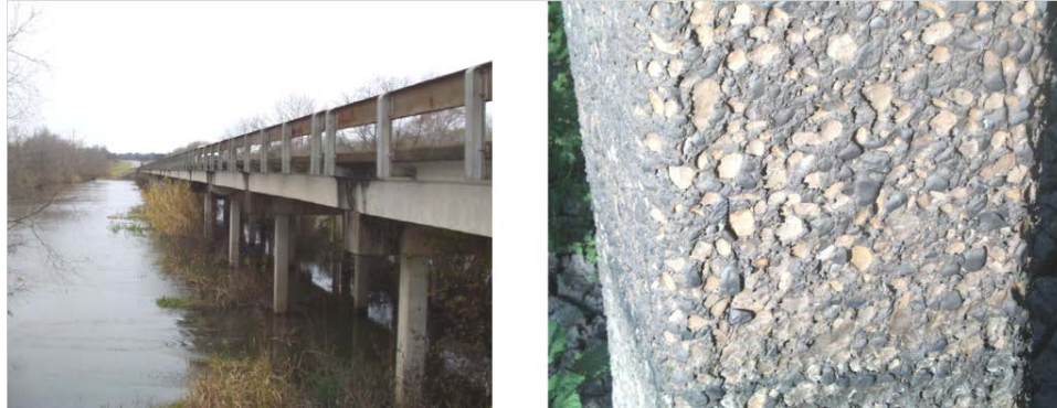
a. Example biodeterioration of concrete surface in Texas bridge structure.
