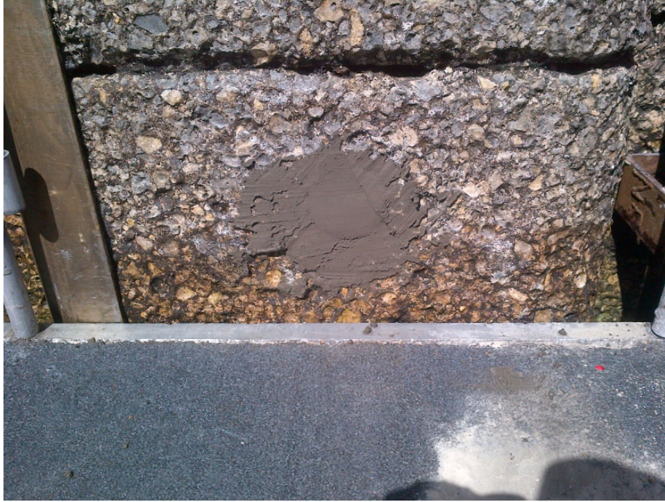
Figure 2. Typical concrete deterioration at location where concrete core was extracted.
