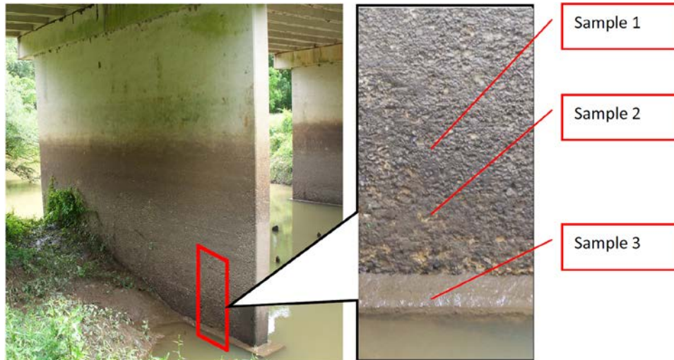
b. Sampling locations for study of surface biodeterioration in Texas bridge structure.
