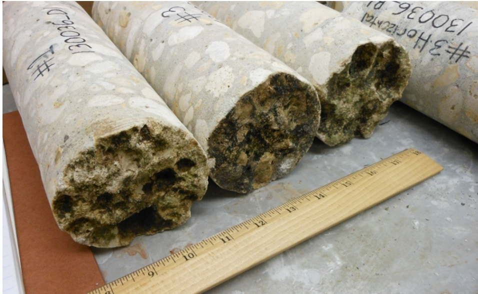
Figure 3. As-received concrete cores from deteriorated areas of S65E.
