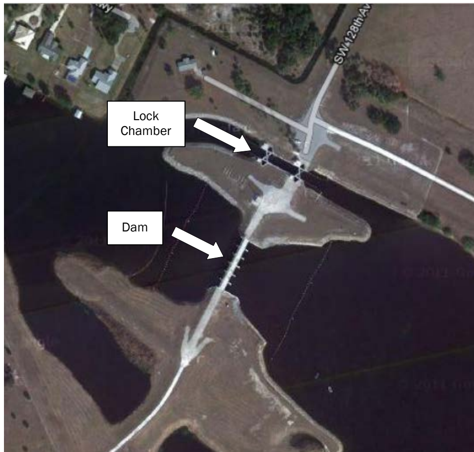
Figure 1. Aerial view of lock and dam structure S65E.
