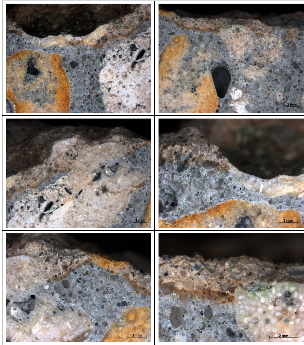
Figure A2. Supplemental photomicrographs of deteriorated concrete from core D2.
