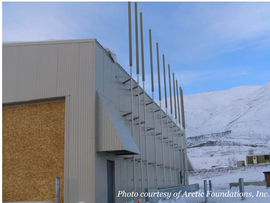
Figure 14. Heavy equipment shop, Chandalar, AK.
