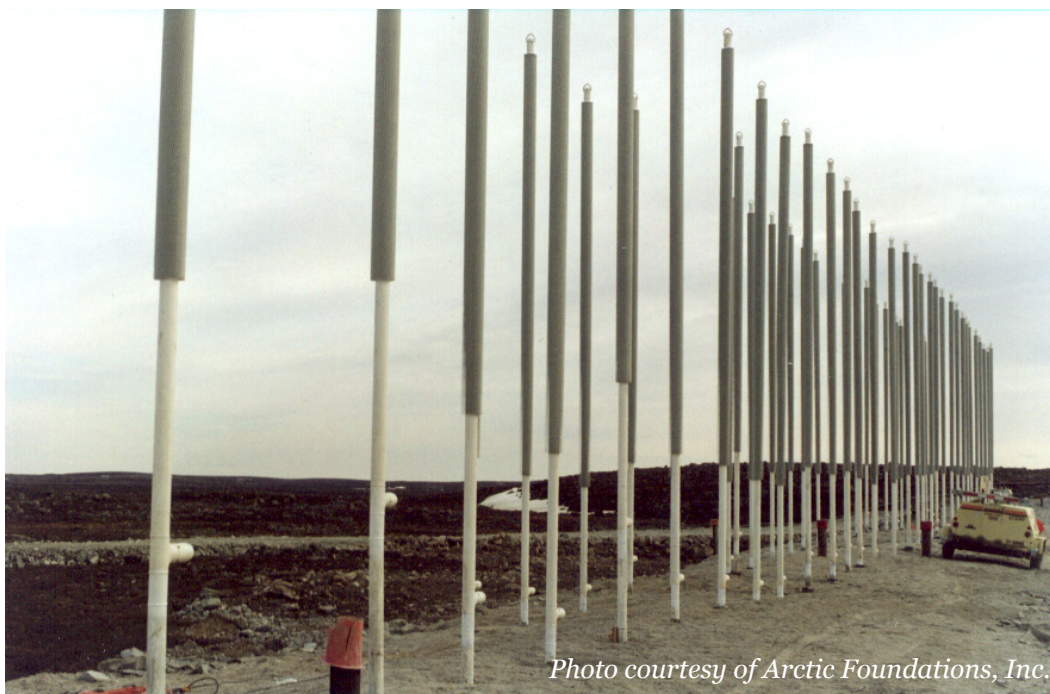
Figure 21. Thermoprobes at the Long Lake Outlet Dam, Ekati Diamond Mine, Northwest Territory, Canada.
