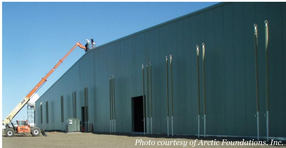
Figure 13. Hangar facility, Deadhorse, AK.
