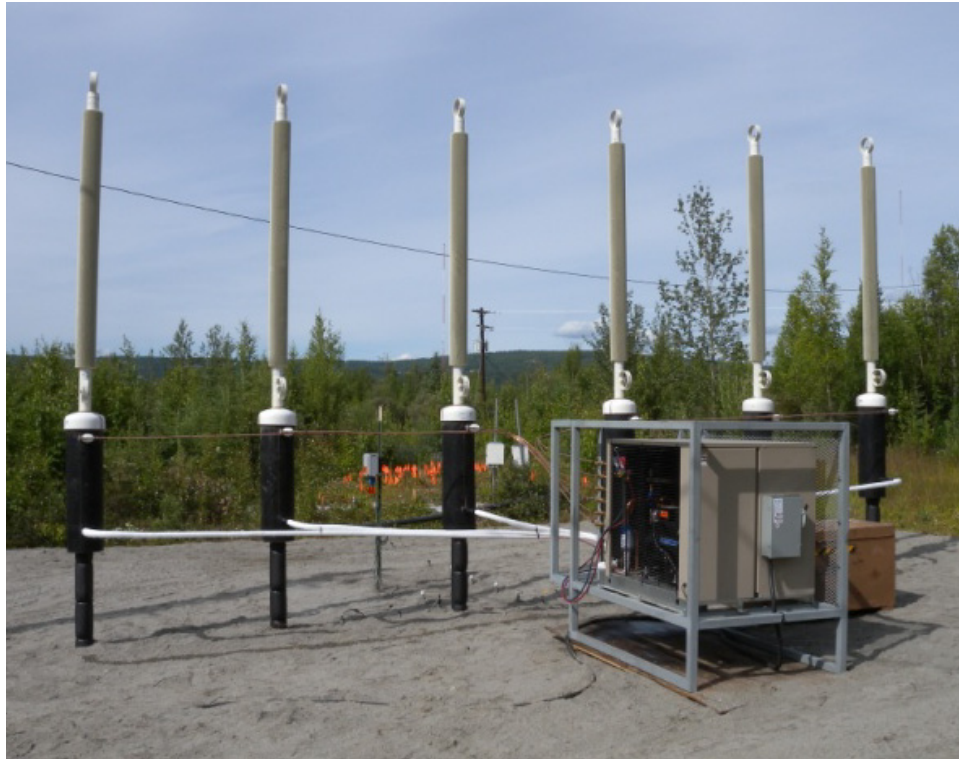
Figure 4. Hybrid thermosyphons installed in Fairbanks, AK.
