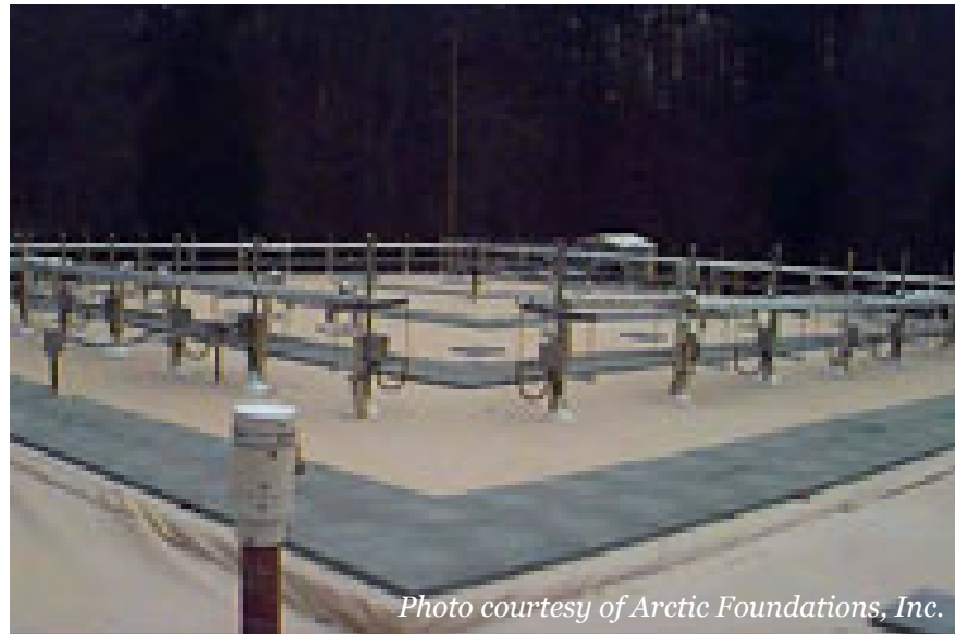
Figure 20. Hybrid thermosyphon system for hazardous waste containment at Oak Ridge National Laboratory, TN.
