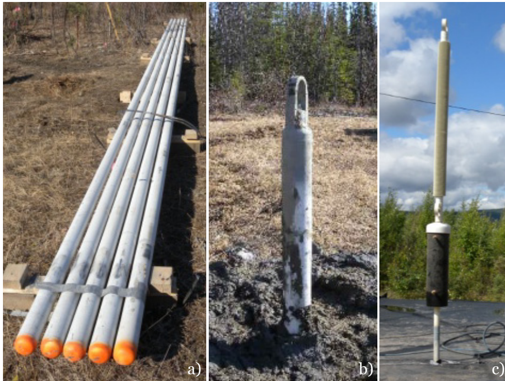
Figure 3. Hybrid system: a) Uninstalled evaporators, b) installed evaporator, and c) condenser.
