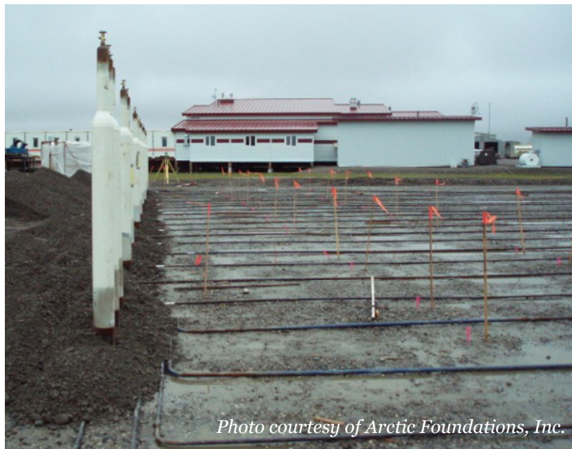
b. Thermosyphons prior to fin installation.
