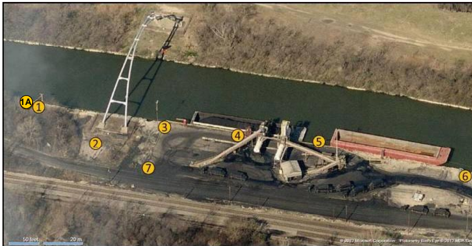
Figure 15. Oxbow Facility with shore measurement test points.
